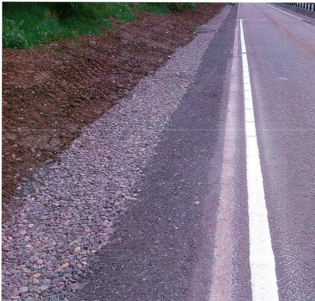
Typical Soft Verge Detail Option 3 (Soft Verge, No Drainage)
